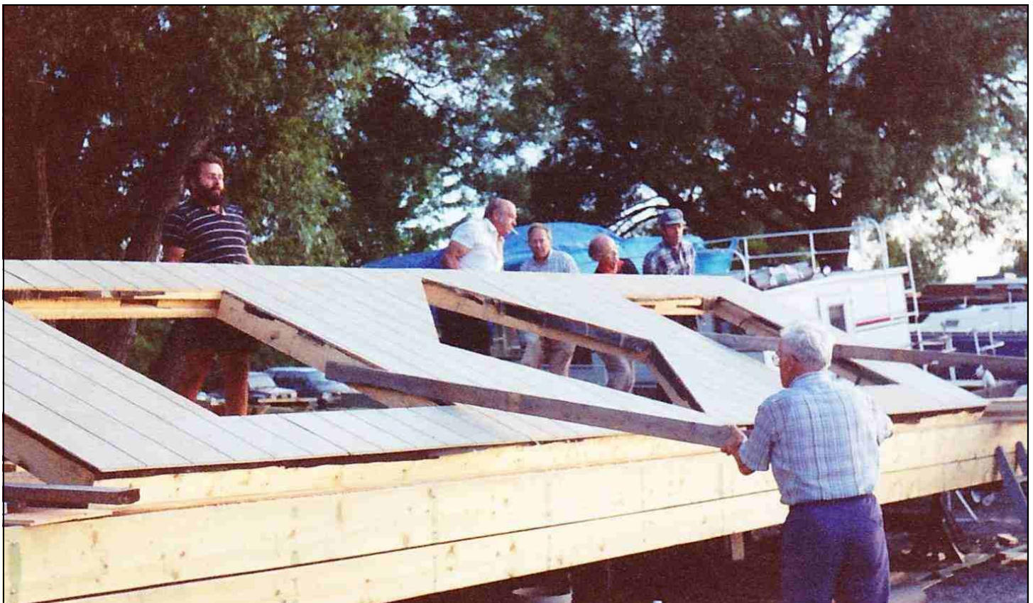
CBYC Members hard at work building the new clubhouse.
